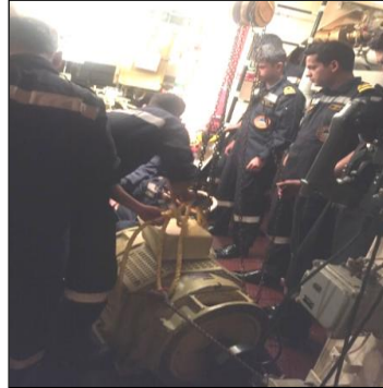
Fig. 2 Lifting of Motor
