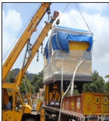
Fig. 11 Installation and Commissioning of 1.5 MW Load Bank
