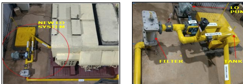
Fig. 10 New Lub Oil System for TBU
